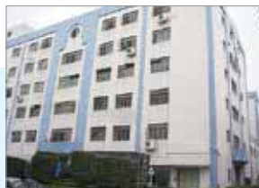
MEAN WELL GUANGZHOU TIANHE R&D CENTER
